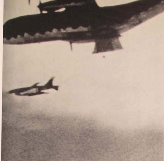
A DC-130 launches a BGM-34A, a specially modified Firebee, with an AGM-65 Maverick . . . it streaks toward the target . . . it approaches . . . and impacts on simulated SAM radar van.
